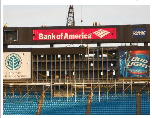
DHG contracted by Turner Construction to provide selective structural demolition during this stadium renovation project. Scope of work included the demolition of the two scoreboards leaving the main structural columns and lower levels only; restroom demolition was included to make way for the new AV room. All of the work was performed 200' above stadium seating and concession stands. Very tight timeframe requiring 7 days a week schedule. Work completed safely and on time.
